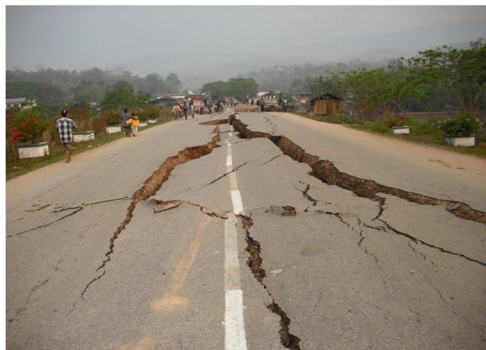
Figure 5. Road collapse due to Myanmar earthquake [13]
