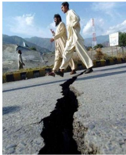
Figure 3. Road damage due to Balakot, Pakistan earthquake [8]
