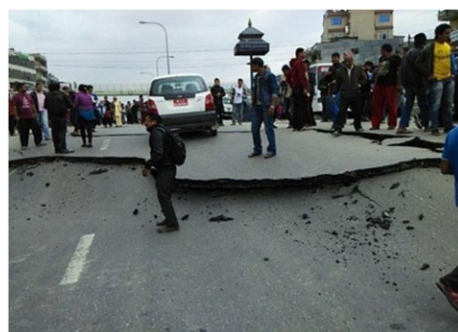
Figure 7. Road damage due to Nepal earthquake [17]
