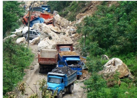
Figure 4. Road collapse due to Wenchuan earthquake (China) [10]
